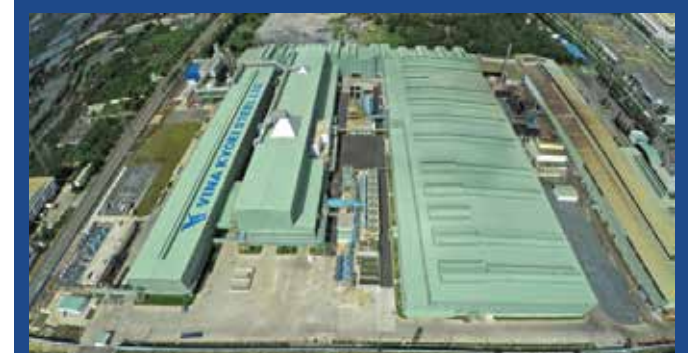
VINA Kyoiei Steel Factory
