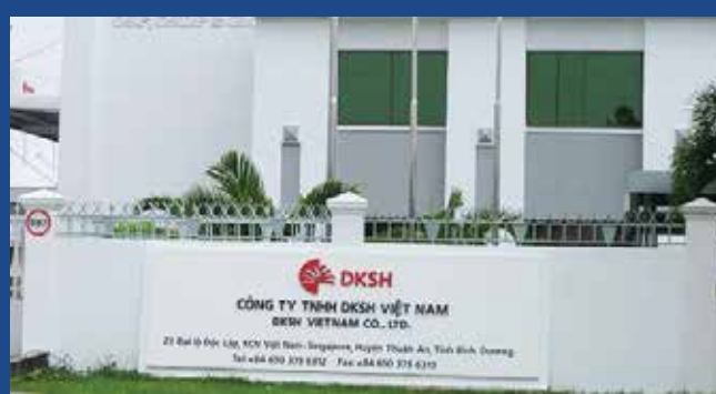
DKSH Vietnam Warehouse
