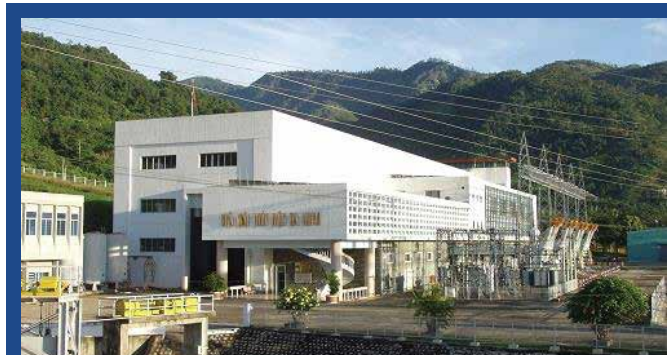
Da Nhim Hydropower Plant
