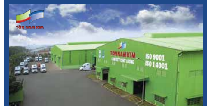
Nam Kim Steel Sheet Factory
