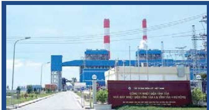
Vinh Tan Thermal Power Plant
